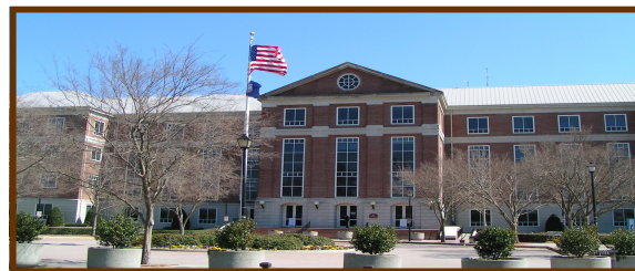
The Virginia Beach Municipal Court Building
